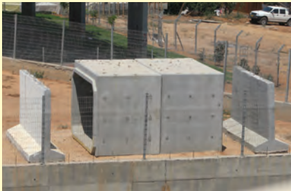
Aboveground bomb shelter on a school playground in Sderot to protect children from the constant rocket attacks from Gaza.
